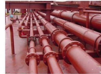
Pipeline Inspection and Maintenance
